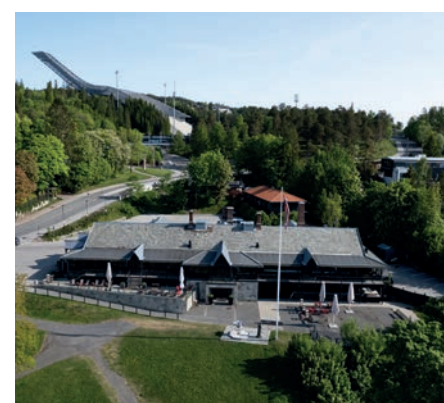
Holmenkollveien 119, Holmenkollen Restaurant 2 100 kvm
